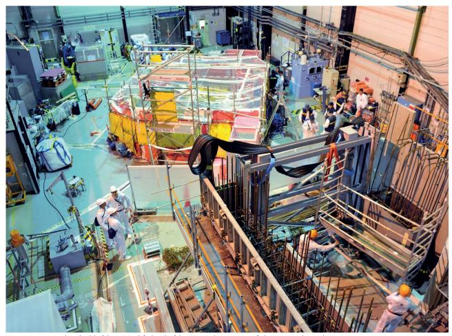
Decommissioning work on the slab of the HAO South facility silo of the UP2-400 plant. Areva spent fuel reprocessing plant on the La Hague site.
