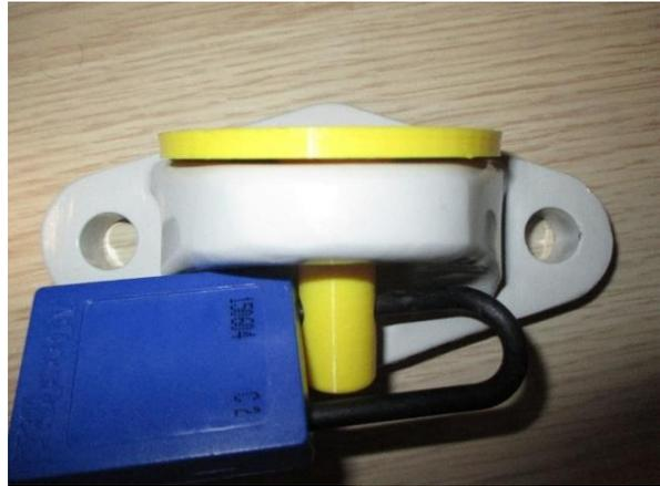
Figure 2: Tagged-out Tie-Off Point
