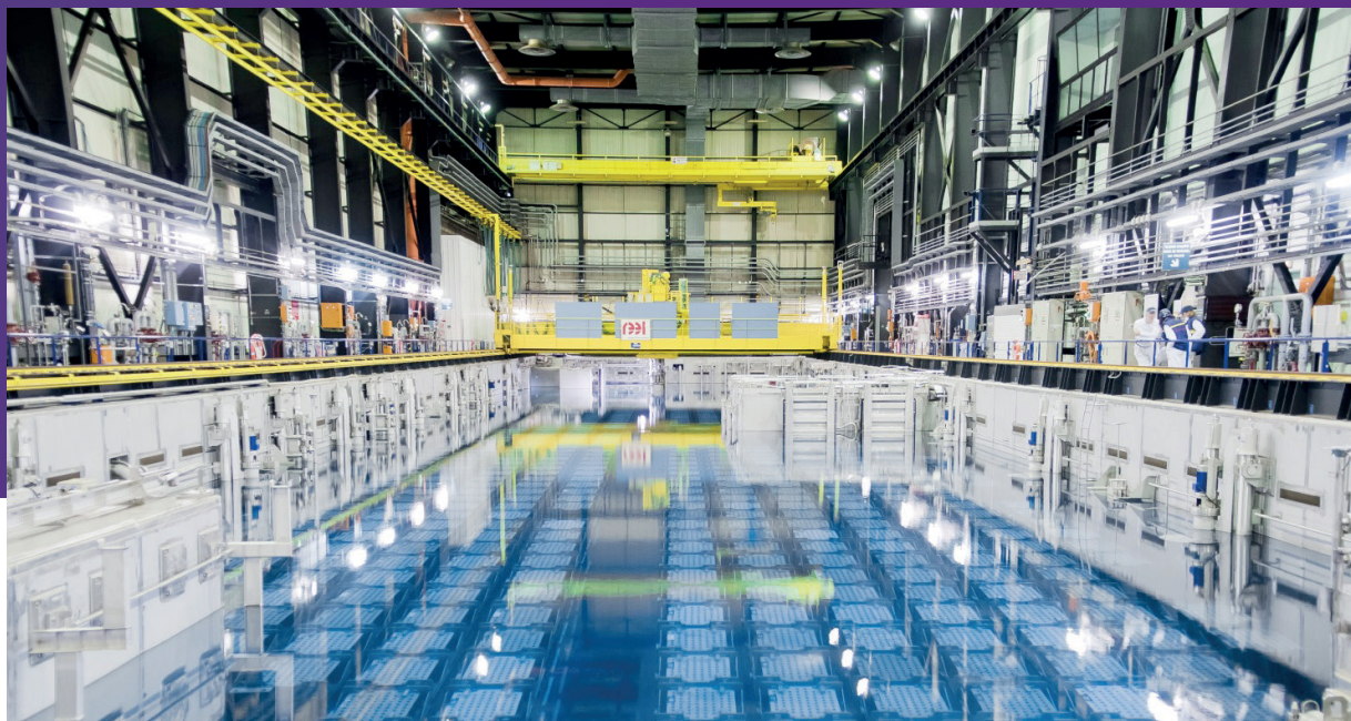
Spent fuel pool at La Hague
