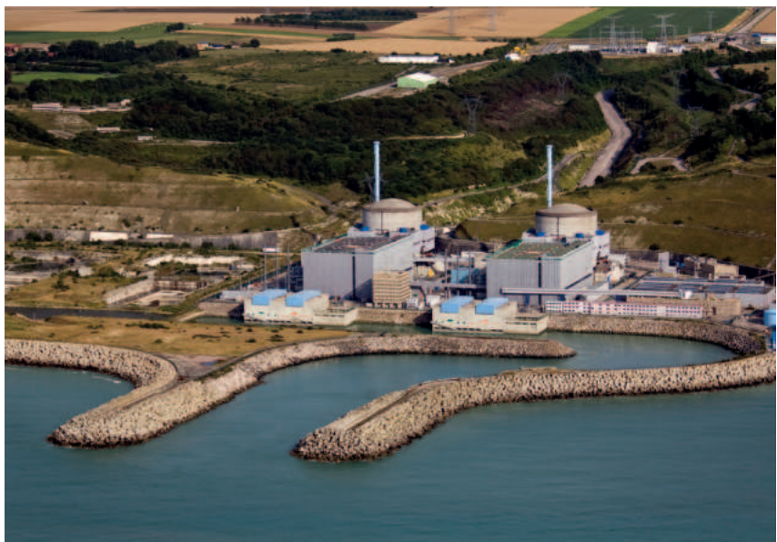
Penly (Seine-Maritime département (1) ) site on which EDF intends to build two EPR 2 type reactors.
