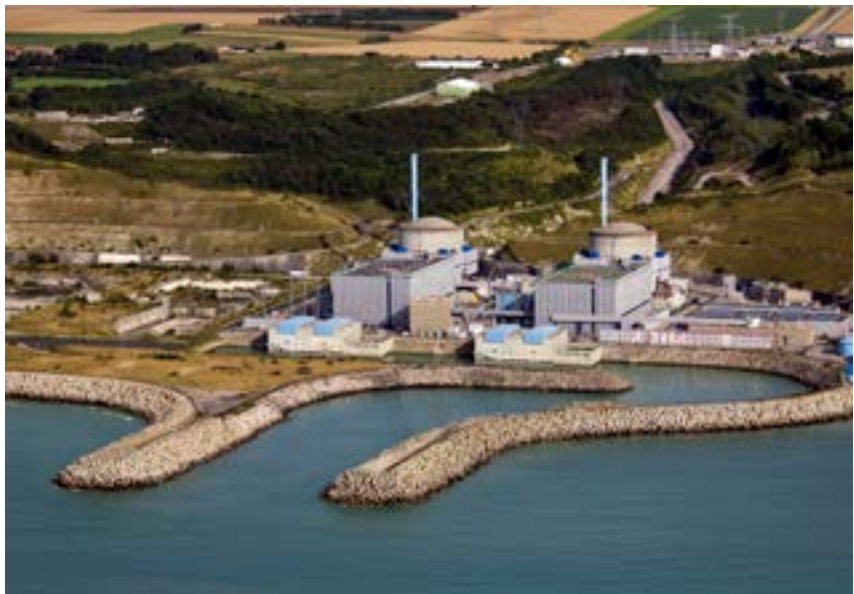
Penly (Seine-Maritime département (6) ) site on which EDF intends to build two EPR 2 type reactors.
