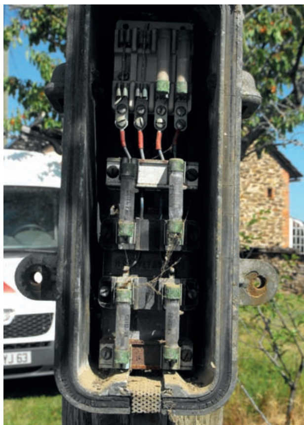
Surge arrester on a telephone line
