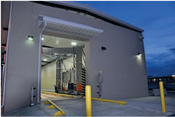
Road freight inspection system
